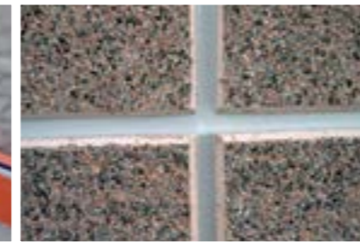
Joints in precast elements
