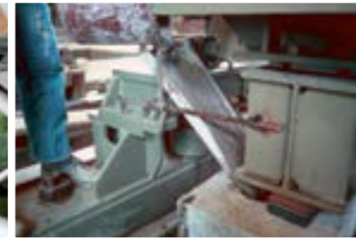
Machine base plate grouting
