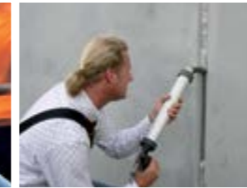
Joint sealing
