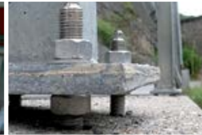
Anchoring; bonding of threaded rods and rebars
