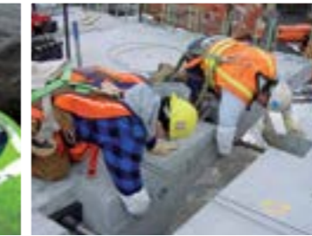
Structural bonding and grouting
