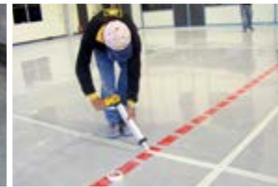
Joint sealing
