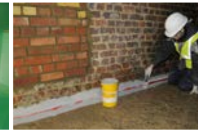
Joint waterproofing
