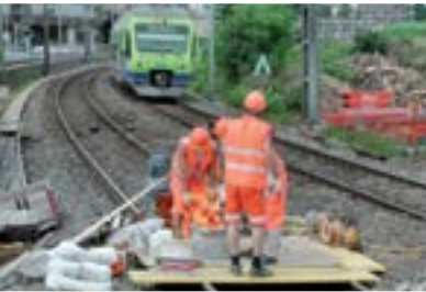
Track/baseplate grouting
