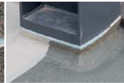
Floor connection joints
