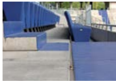
Floor movement joints
