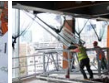
Steel and glass façade
